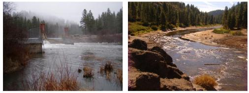
**Figure 2.** Chiloquin Dam from downstream prior to removal (left) and post removal (right).
